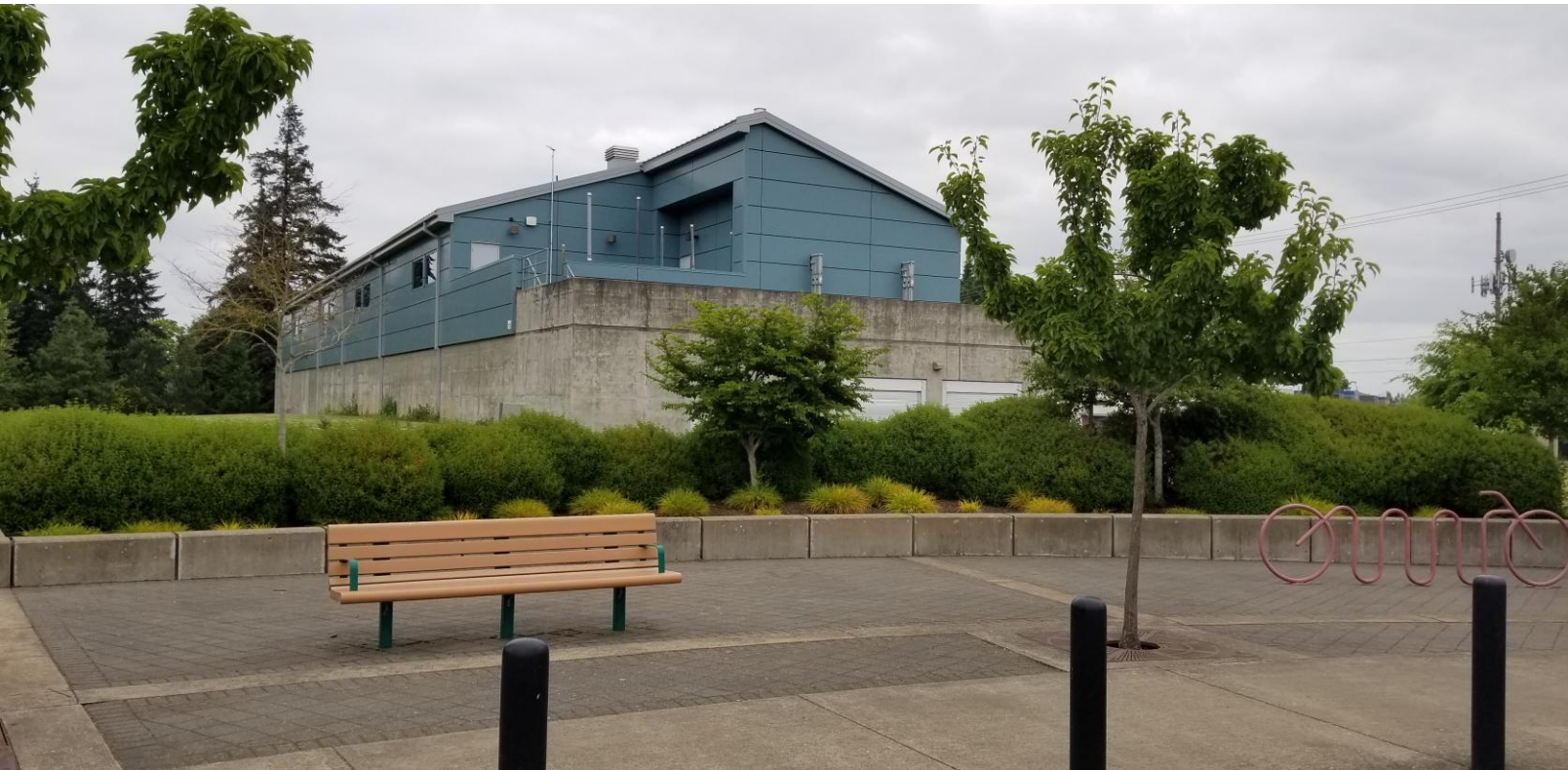
River Road Park and Wet-Weather Treatment Facility
